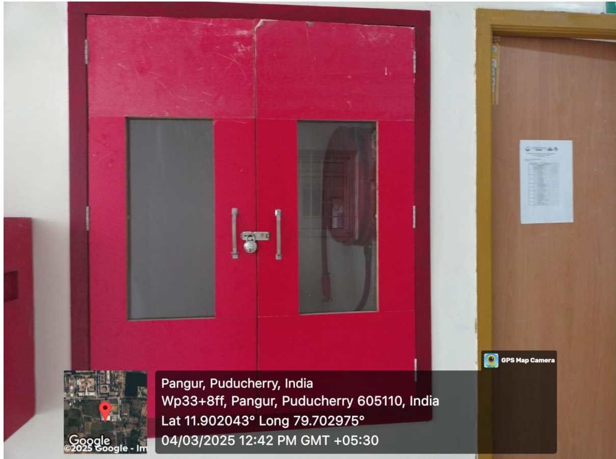
Figure iii: Fire Hydrant System
